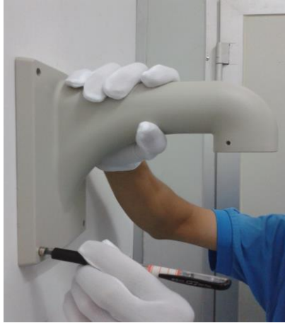
picture 3-4 Determine the screw holes position
